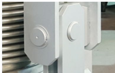
PTFE bushes on the anchorages minimize friction and thus adjustment forces
